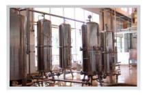
**Lenticular Modules Housings** These housings are manufactured with highly resistant materials that guarantee optimal performance of the filtration elements.
